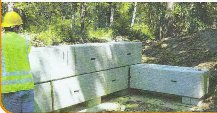
Preparing foundations and setting first row of blocks
