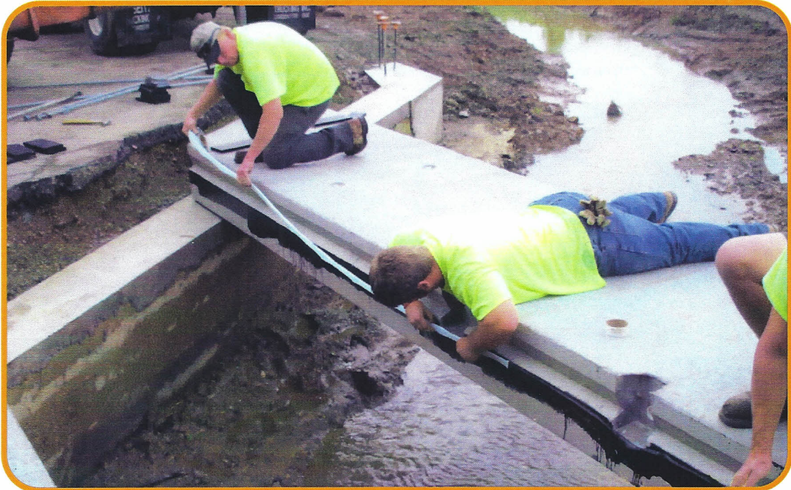
Beams being set on reconditioned existing abutments
