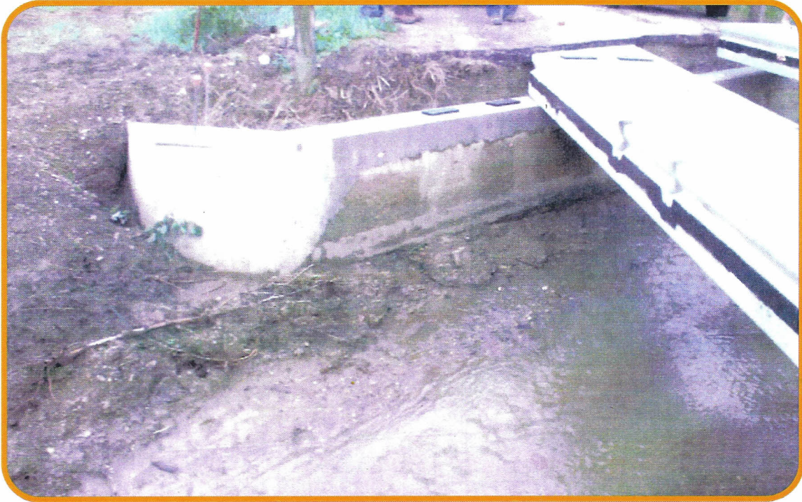
Beams being set on reconditioned existing abutments
